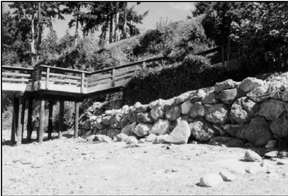
Figure 2. Rock bulkhead constructed on shore south of pier.
