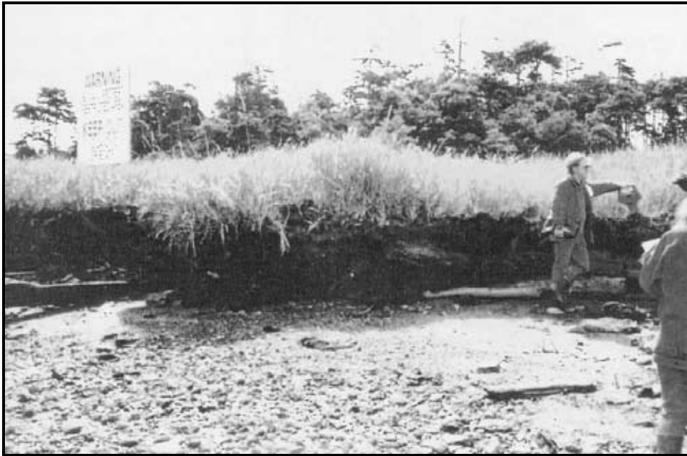
Photo 3. Erosional scarp in bank prior to construction, exposing waste from former landfill ( Photo: courtesy of Bill Kalina, Navy ).
