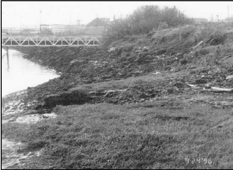
Figure 1. View south of site prior to construction. Note vegetated upper intertidal benches.
