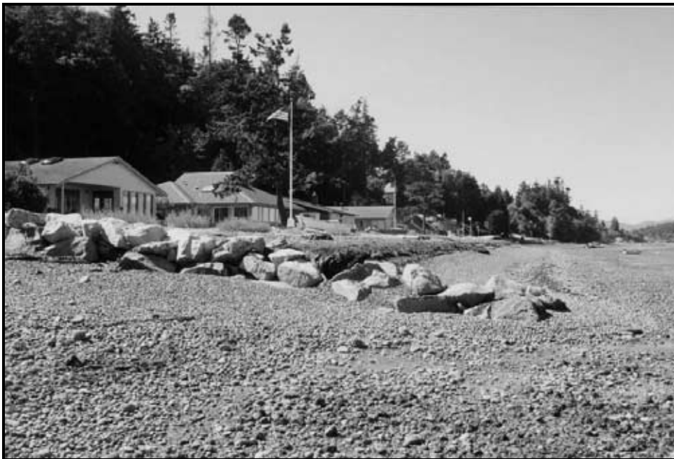
Figure 2. Looking west at project, including drift sill (groin) that forms eastern end of nourishment. Note that beach is considerably lower on east (left) side of structure. It is important that gravel be able to continue to bypass the structure in order to feed downdrift beaches.
