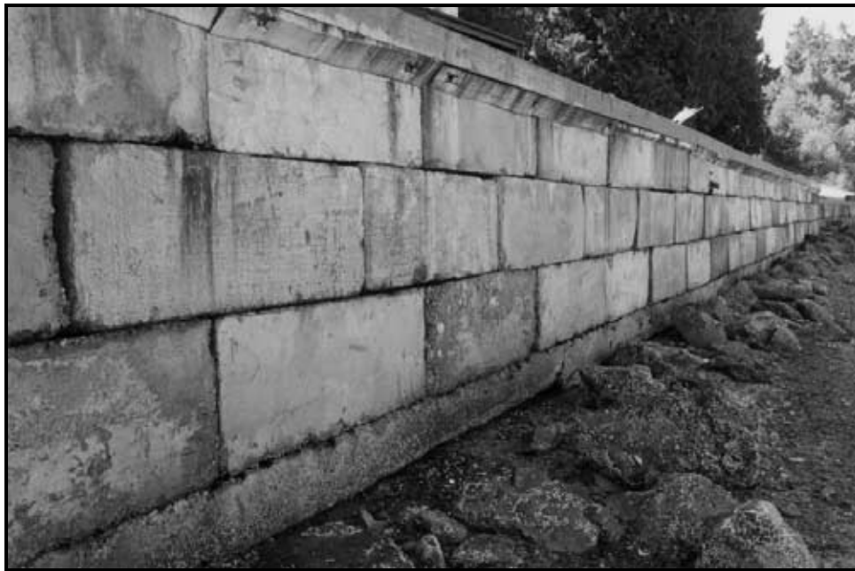
Figure 4. Ecology-block bulkhead located immediately west of project area.. Riprap has been added to protect base from scour.
