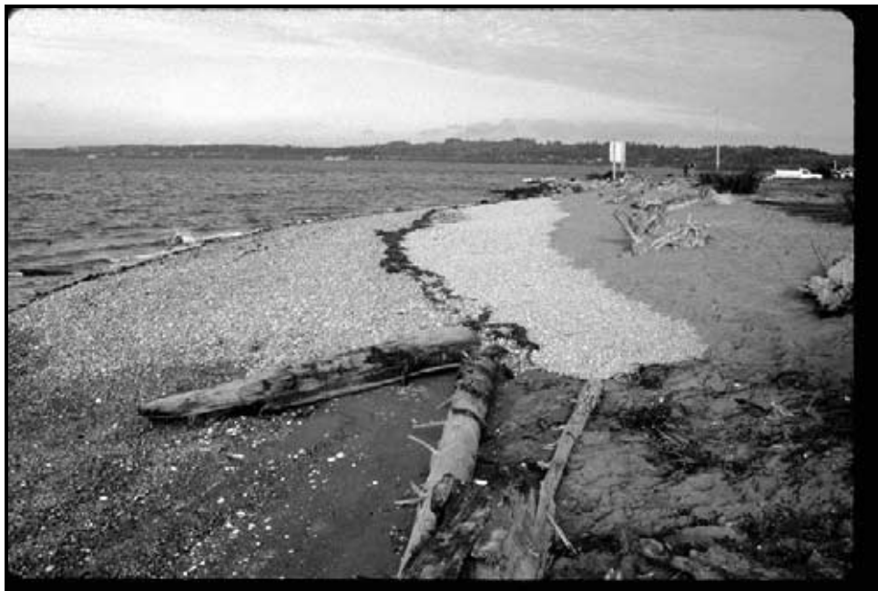
Figure 4. View to the east immediately following construction (Fall, 1995), showing gravel beach and recent high tide line. Note sand placed on landward portion of the berm.
