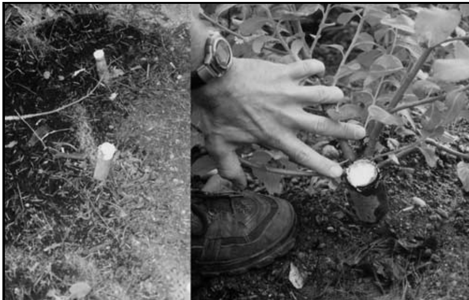
Figure 4. Live staking. When willow stakes are installed there is no growth - just a 1.5" portion of a 2-foot stake driven into the substrate. Four months later, vigorous growth has begun to secure soils in place.
