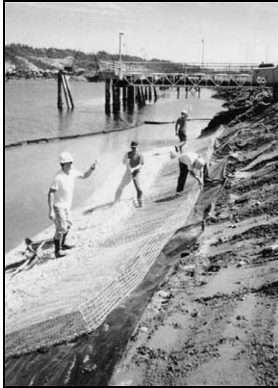
Figure 3. Installation of gabion mattresses over geotextile ( Photo: Joyce Mercuri )
