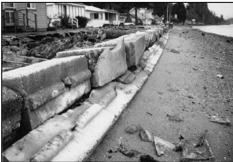
Figure 6. Ecology-block wall prior to nourishment. Failure occurred in the winter of 1996-1997 by undermining and excess hydrostatic pressure - upper tier has been restacked in this photo. Note erosion of upland area behind wall.
