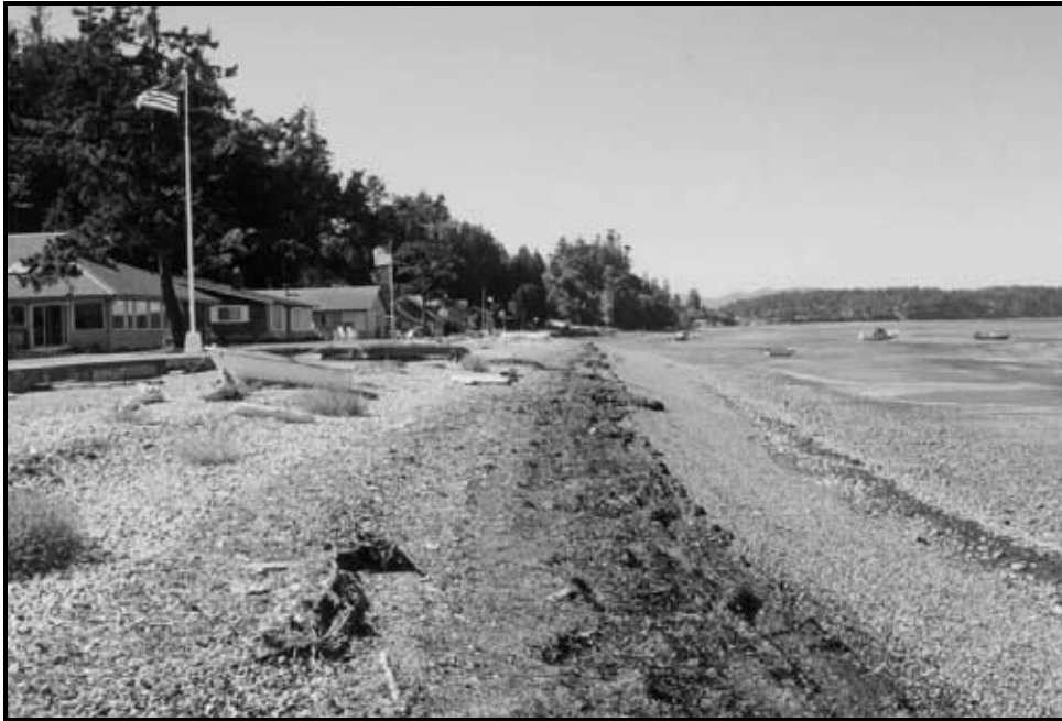
Figure 1. View west from the east end of the project. Note broad gravel berm and recent accumulation of beach wrack. Prior to nourishment, the bulkheads at the left were in danger of undermining.
