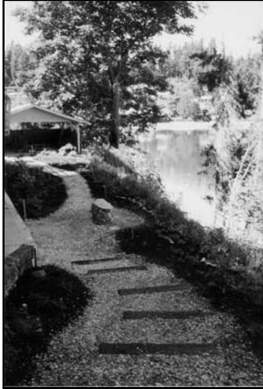
Figure 3. Path in front of house. Prior to construction this was part of the driveway, but narrowing the path allowed more room for laying back the slope.
