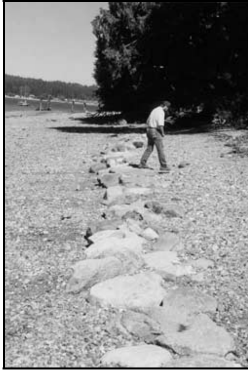
Figure 3. This row of boulders was placed to help stabilize upper portion of gravel beach.
