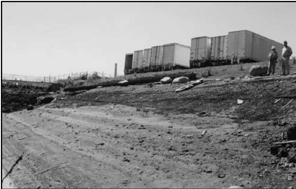
Figure 2. View southwest of site after construction. Fine sediment covers gabion mattresses except in area immediately below bench (people standing).
