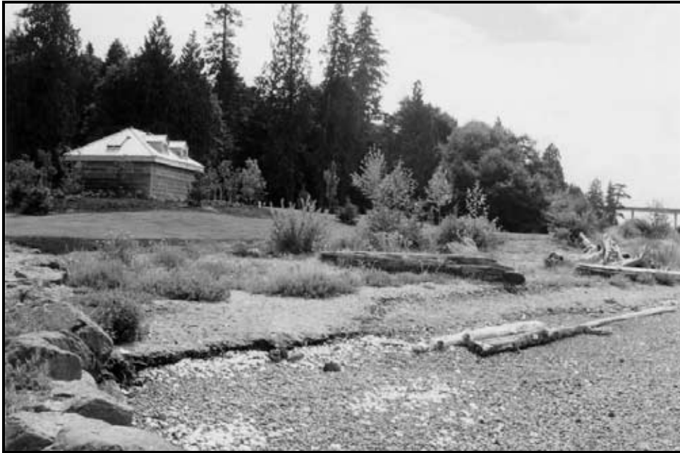
Figure 1. View west showing gravel beach and backshore. Large logs in the backshore were placed at construction, whereas most vegetation has reestablished naturally (1999).
