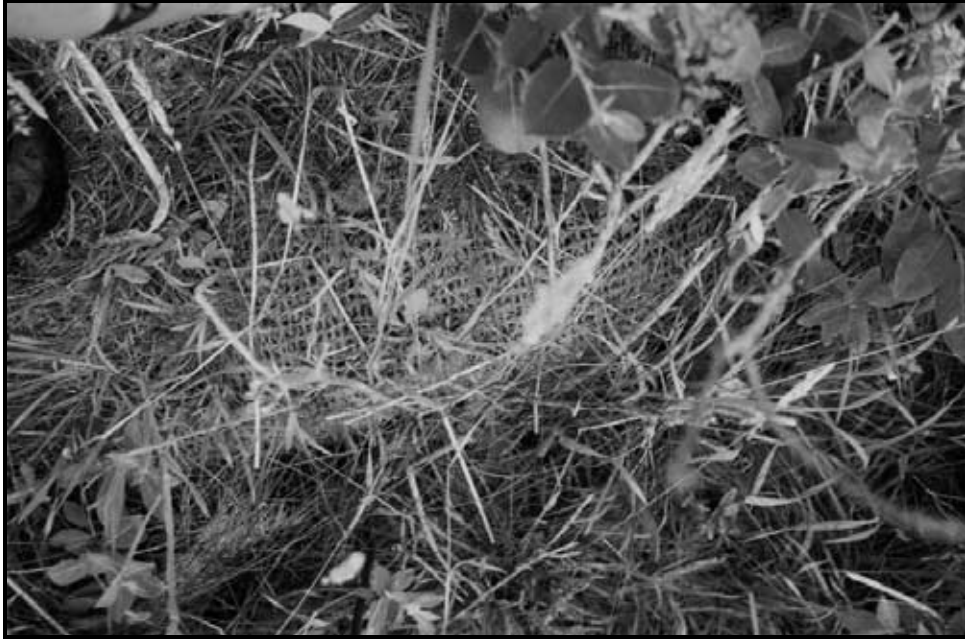
Figure 5. Natural fiber geotextile. Coir fabric is exposed on the face of a geogrid lift.
