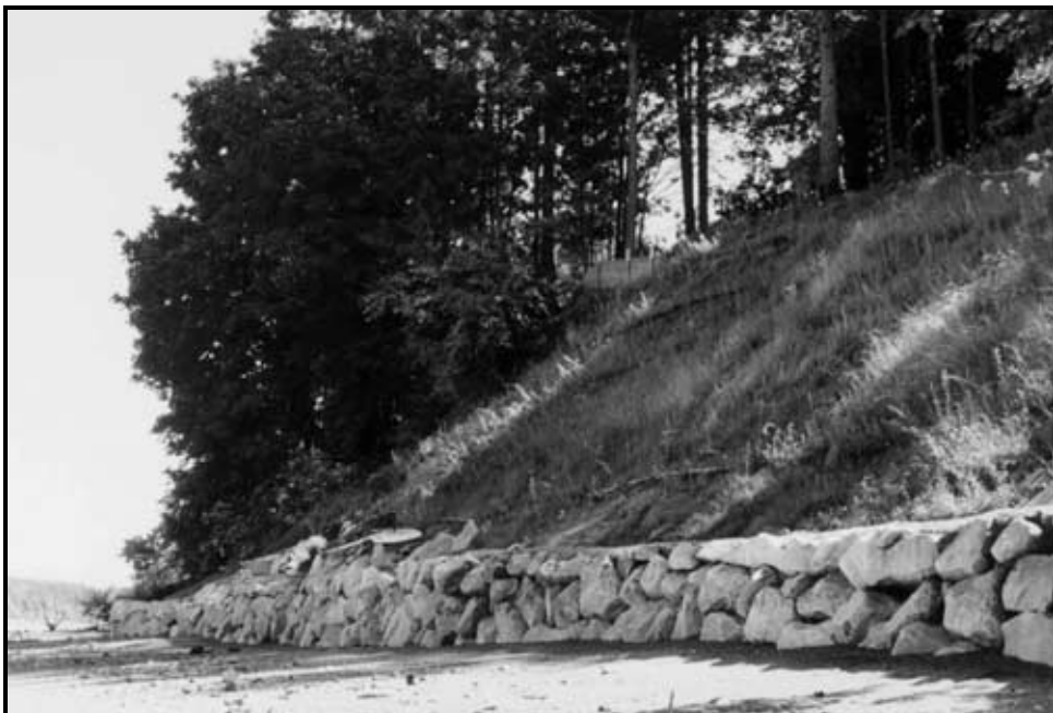
Figure 2. View from the beach. The lift layers can be seen. The slope is approximately 1H:1V, compared to its original near-vertical pre-construction state. The bluff is 30+ feet tall (the rock bulkhead is 5-6 feet high).
