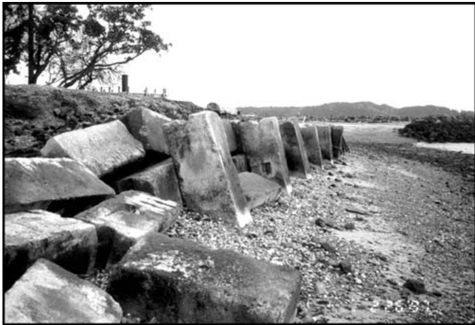
Figure 2. View northwest showing temporary "ecology block" erosion protection. Note significant damage done to temporary structure. Breakwater for boat basin is in background.
