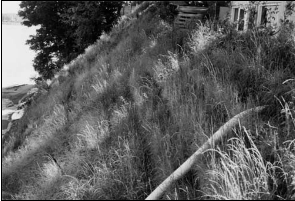
Figure 1. Vegetative slope stabilization. The bands of vegetation correspond to individual geogrid lifts. The hose in the foreground is part of new drainage system and flows into a diffuser behind the bulkhead.
