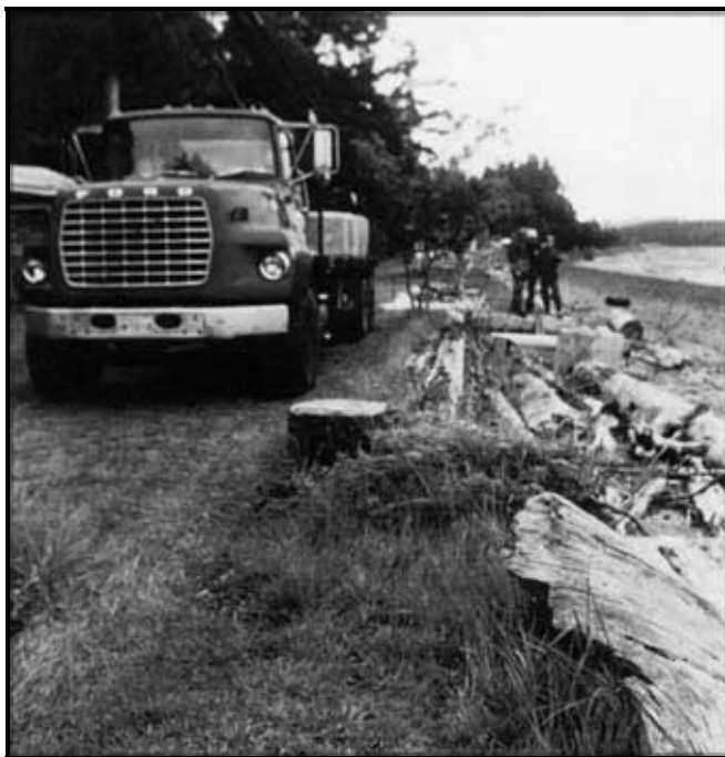
Figure 5. Photo taken immediately prior to bulkhead construction in 1982 along east-central portion of project site. Note line of drift logs and narrow berm (Photo: courtesy of Marge Dunnington)
