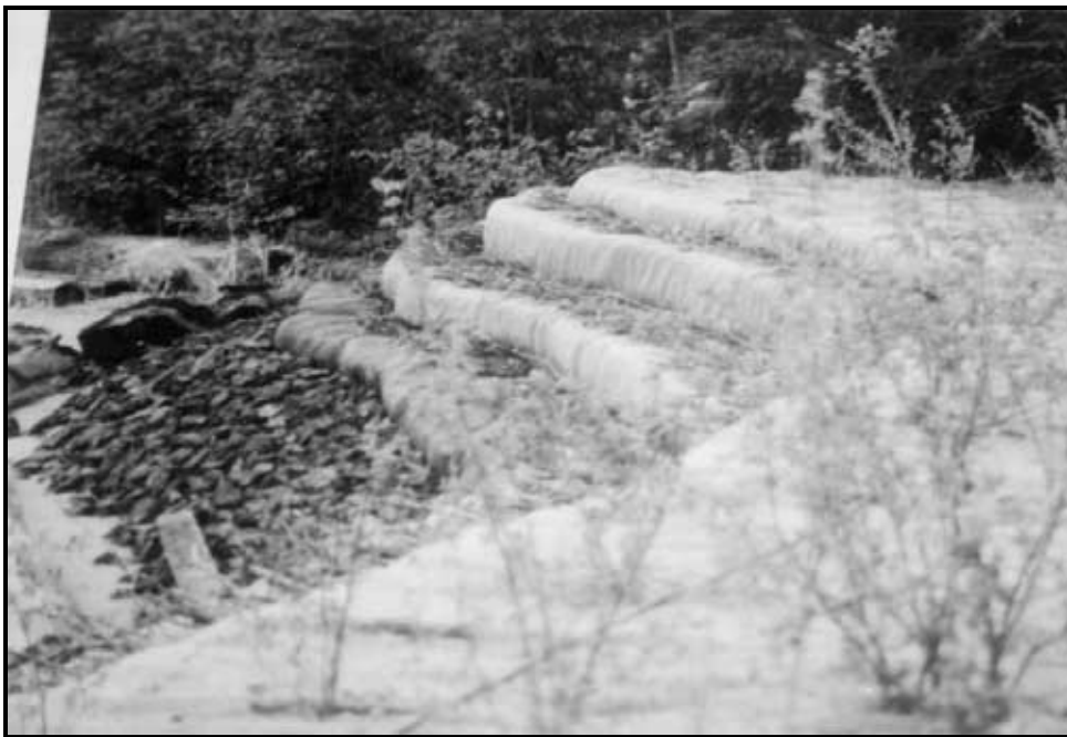
Photo 4. Geogrid lifts are obvious immediately following construction. Geotextile fabric completely covers lifts, but was quickly obscured by vegetation ( Photo: courtesy of Bill Kalina, Navy ).
