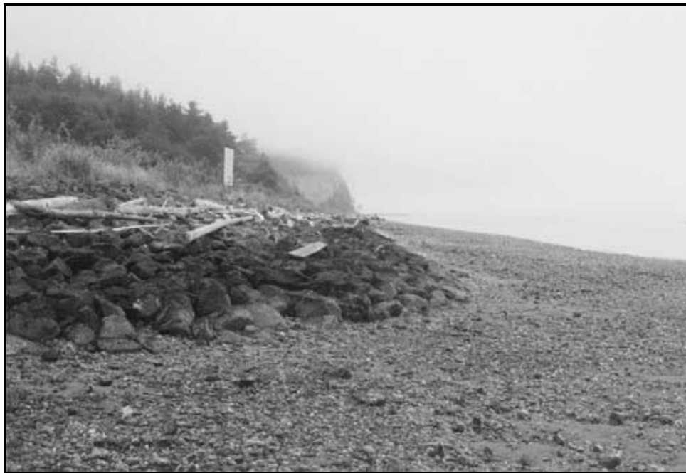
Photo 2. View southwest from northern end of project. A rock revetment is used in the high energy zone.
