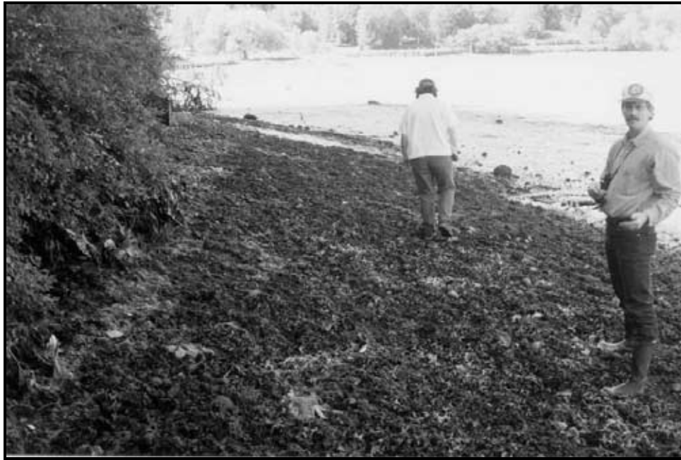
Figure 1. Gravel beach and vegetated bank. Quarry spall was placed at the toe of the slope and is largely covered with gravel. Aquatic vegetation is colonizing the coarse gravel, which is relatively stable in this low energy environment.
