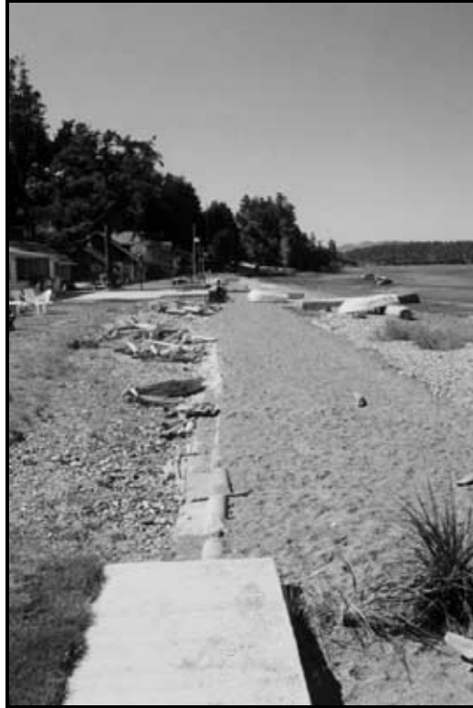
Figure 3. View west along bulkhead line in central portion of project. The bulkhead in the foreground failed in the winter of 1996-1997 (see Figure 6). Note elevation of backshore and placement of sand to facilitate revegetation.
