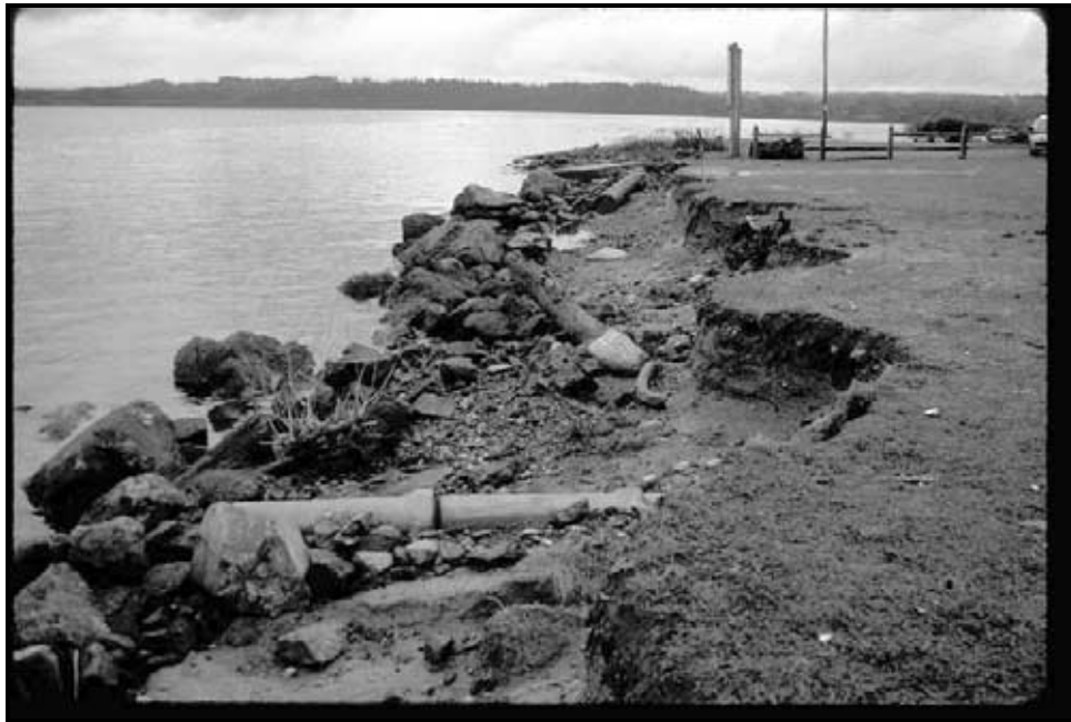
Figure 3. View east of project area prior to nourishment. Note scarp in eroding artificial fill and rocks placed in effort to reduce erosion (1995).
