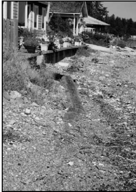
Figure 3. View of east end of site following completion of project. The logs rise out of beach and curve back to meet neighbor's bulkhead.
