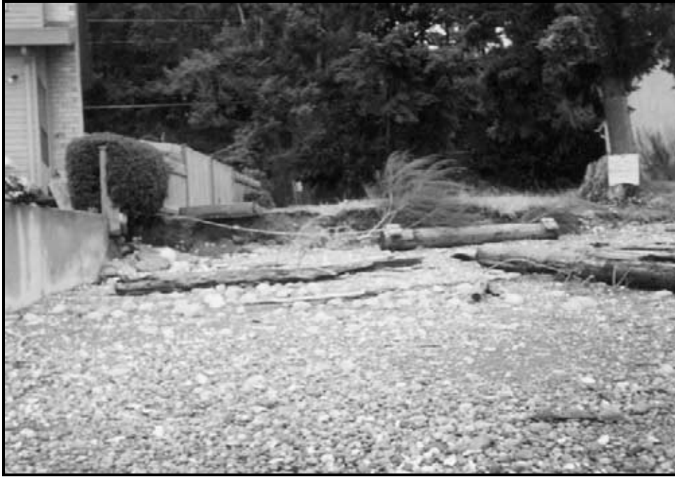
Figure 1. West end of site prior to construction. Note significant scarping and the amount of the neighboring bulkhead's wing wall that is exposed.
