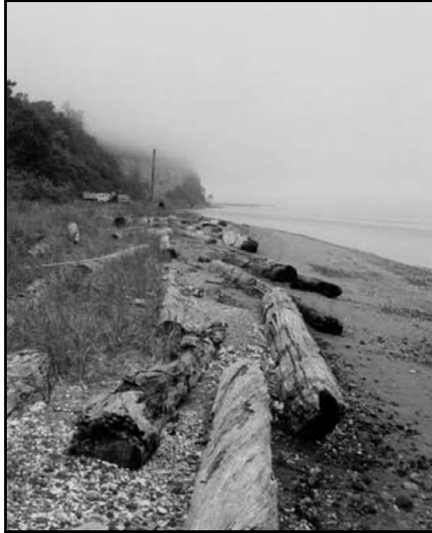
Photo 1. Low energy zone. Coarse woody debris anchored to the beach, with vegetation planted on berm between upper logs.
