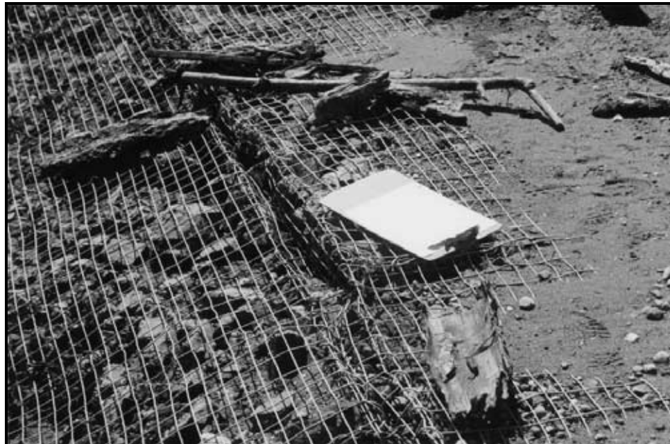
Figure 4. Detail at waterward edge of bench showing exposure of gabions.
