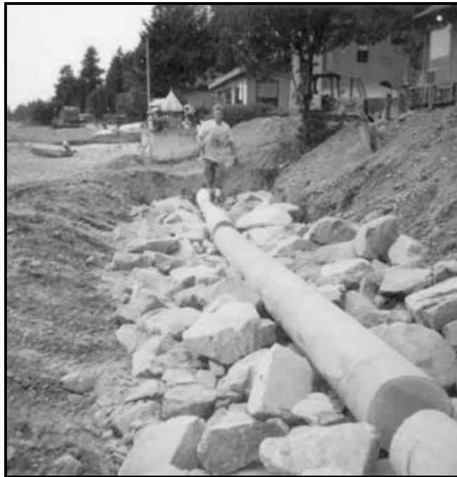
Figure 2. View of west end of site during construction. Large amount of rock provides an emergency bottom in the event that the beach drops ( Photo: Jim Brennan ).
