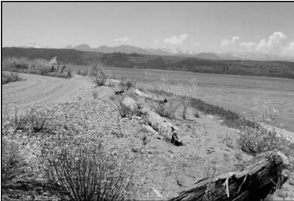
Figure 4. Slope and backshore with road. The position of the road affected the overall design of the project and the grade chosen for the upper beach.
