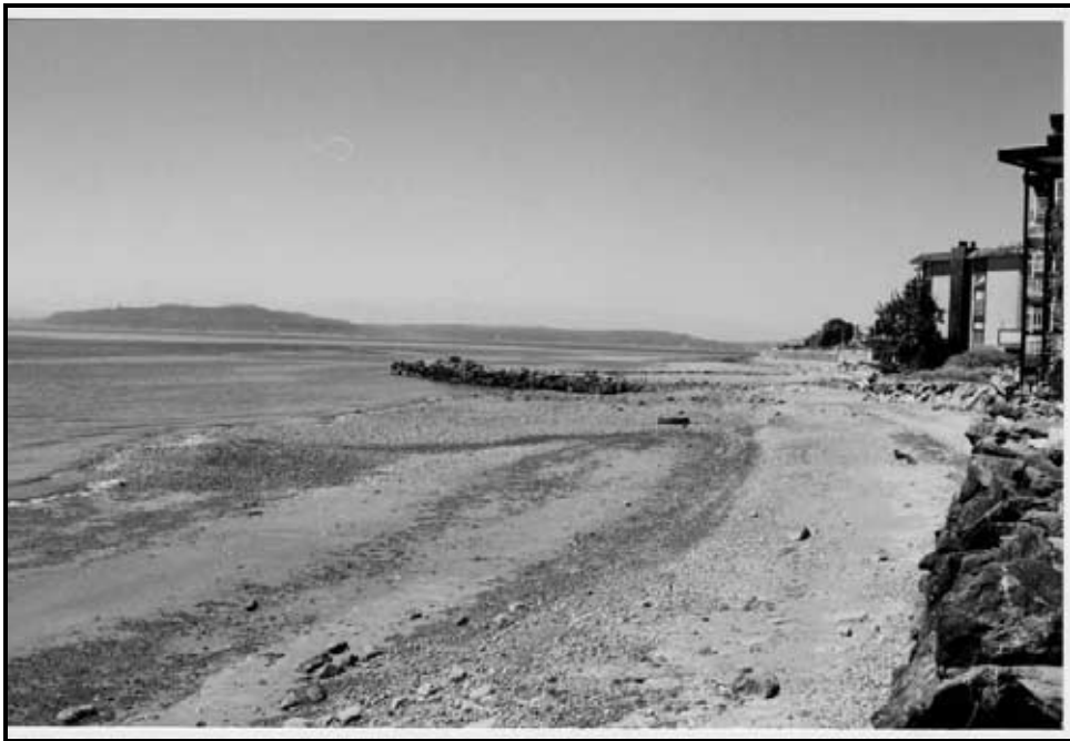
Figure 2. View to the north from 3701 Beach Drive, showing hardened shoreline and intrusion of bulkhead onto upper beach.
