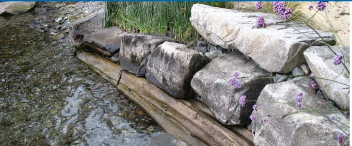
Logs must be anchored securely in place. Although the dense, weathered wood used for these projects does not float easily, a little buoyancy can be enough to pull a log loose during a storm. A loose log can be hazardous to people, structures, or boats. There are several ways to secure a log, but it is most commonly done using duckbill anchors and cables or by partially burying the log.
